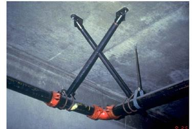
Proper bracing at change in direction
