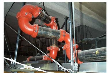
Seismic separation assembly
