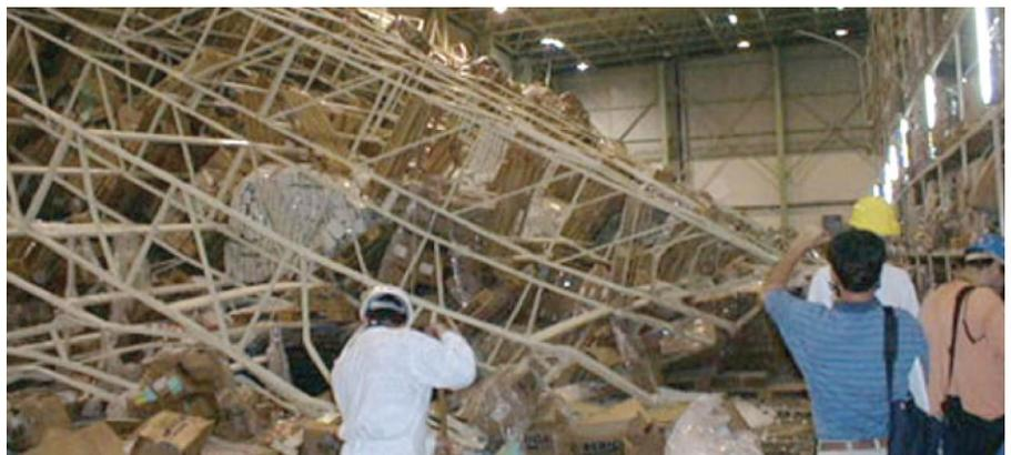
*A high percentage of Turkey's industry is located in the northwestern part of the country near Izmit, the location of a magnitude 7.4 earthquake in August 1999. Toppling of storage racks in this pharmaceutical plant is one example of the substantial damage to industrial facilities that can result from ground shaking.*
